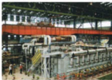
Furnace area in new rebar mill, Jamshedpur
