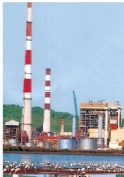
Tata Power facility at Trombay High
